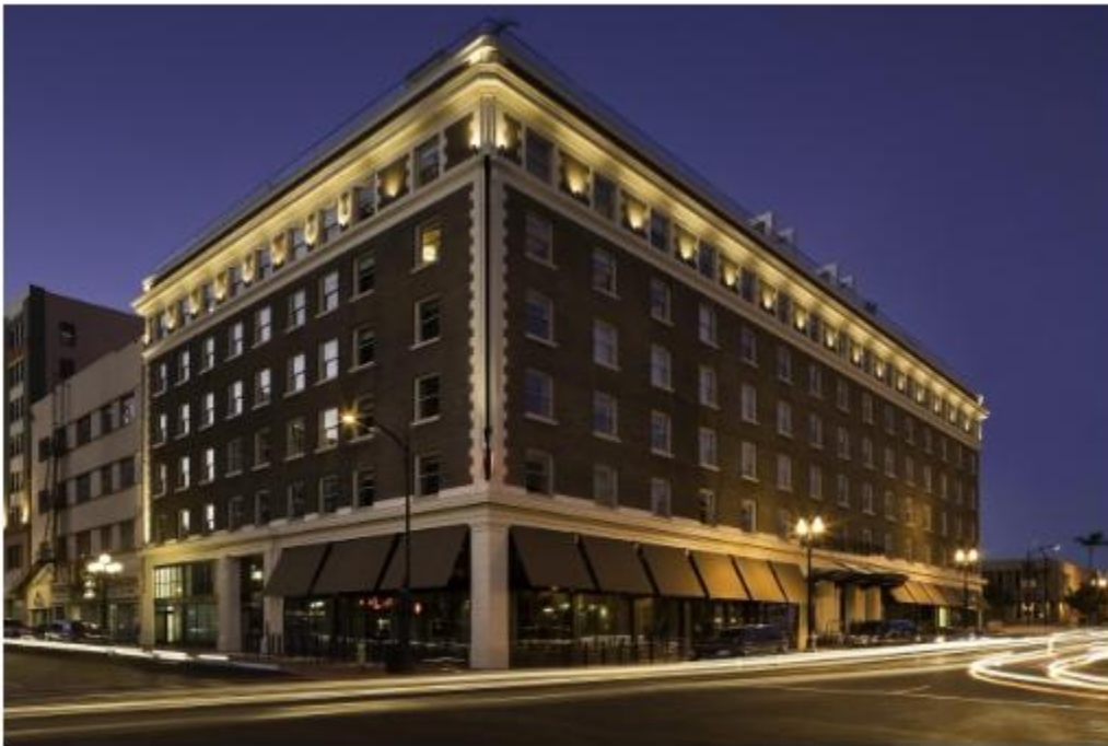
Historic brickfront exterior of the Andaz hotel. Photo: courtesy Andaz hotel
